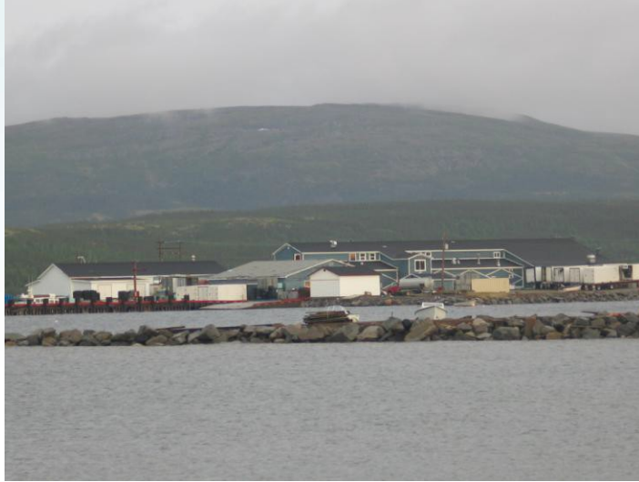
Figure 1: The processing facility in Makkovik.
